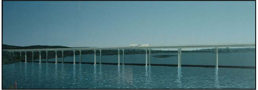
Precast Segmental Bridge, 1st of its kind on the PA Turnpike
