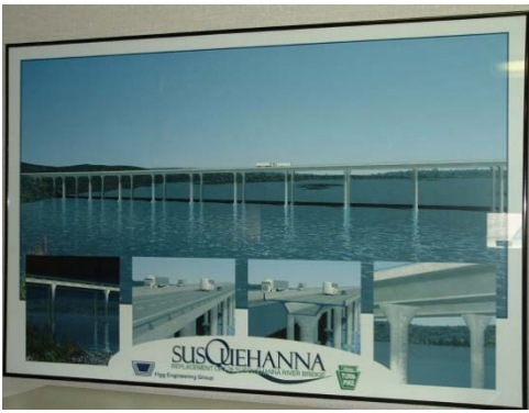
Precast Segmental Bridge, 1st of its kind on the PA Turnpike
